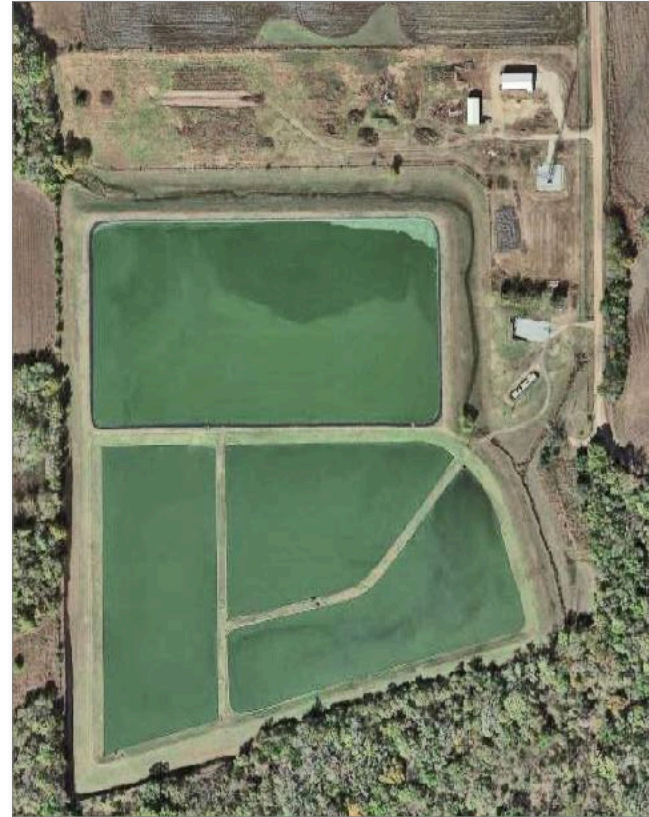
aerial of Clearwater's Sewage Treatment Plant & Lagoons
