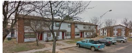
Mimosa Arms — 30-unit low income apartment complex
